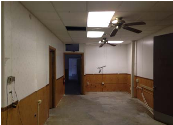
EXTERIOR AND INTERIOR OF EXISTING POLICE DEPARTMENT HEADQUARTERS
