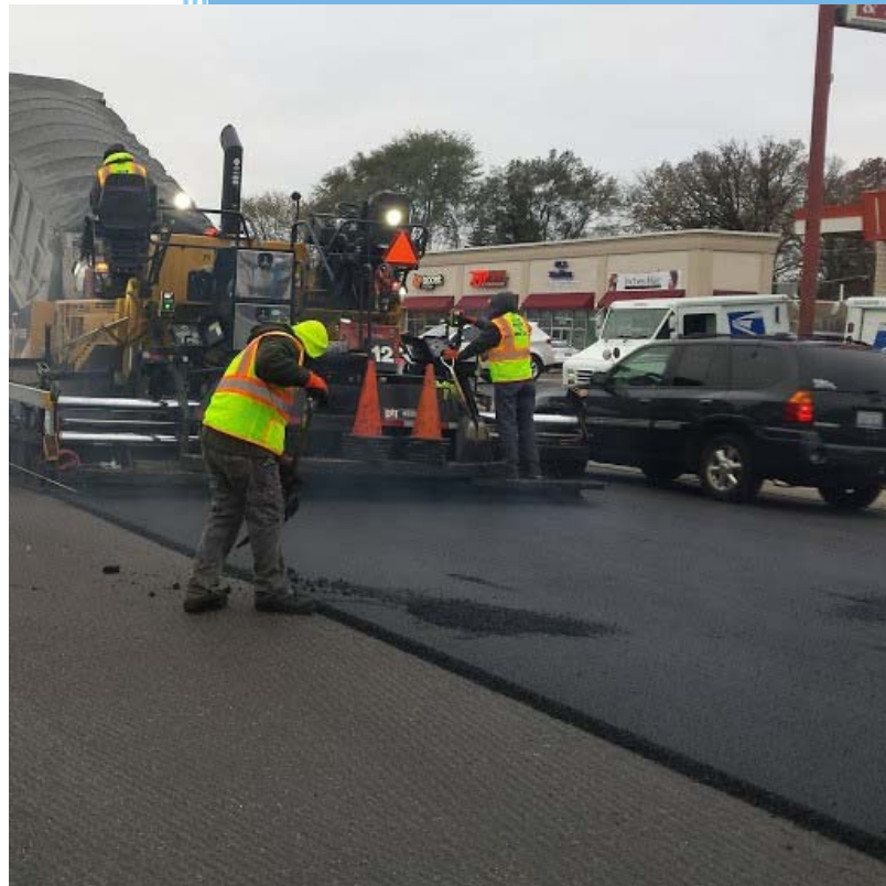
ROAD PAVING PROJECT. WKGN PR DEPT PHOTO CREDIT.
